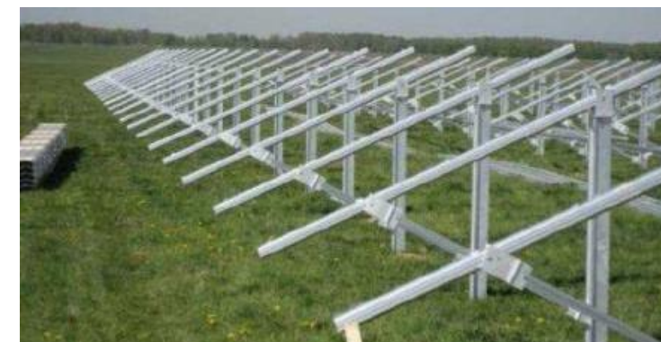
Photo 1 : Structures de support sans modules
